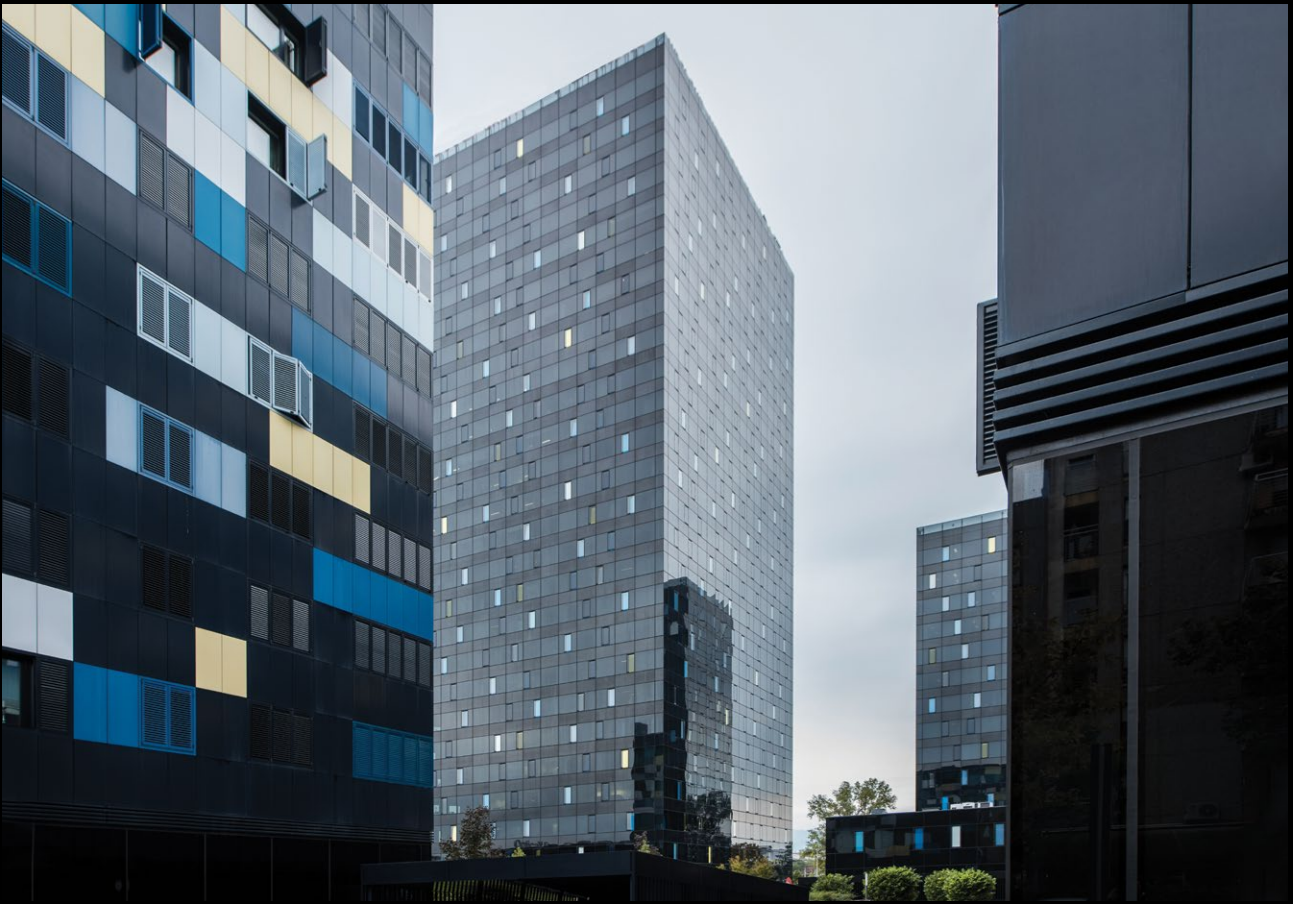
Strojarska Business Center | architecture: Davor Mateković, Tomislav Stojan, Mirna Melez, Ida Ister, Vedran Pavličević
